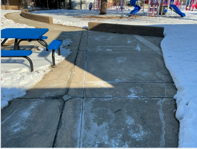
ACCESSIBLE ROUTE TO PLAYGROUND
