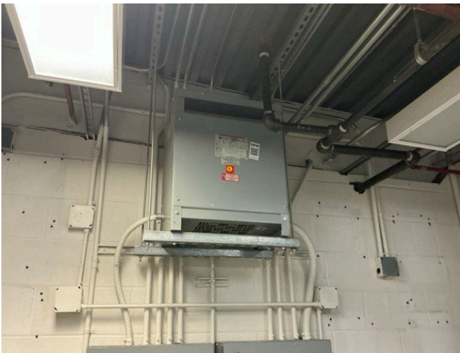
33 - SECONDARY TRANSFORMER
