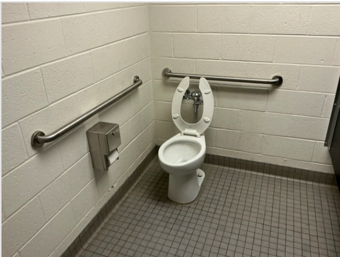
TOILET STALL OVERVIEW
