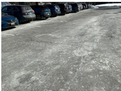
Several alligator and large cracks. POC reports that parking lot floods continuously - AssetCALC ID: 10292111
