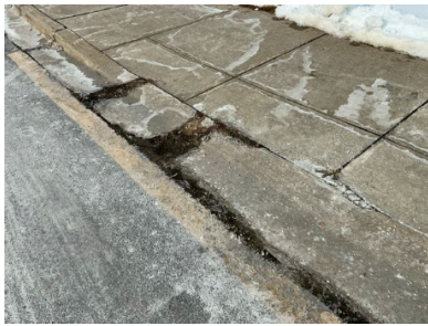
Broken and cracked curb - AssetCALC ID: 10294880
